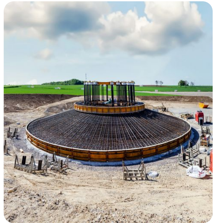
Wind turbine foundation
